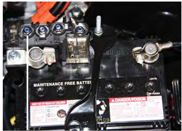
DC to DC Converter Cable Connection
