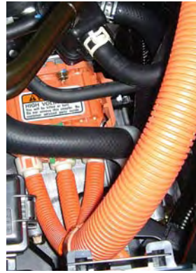
High-Voltage Cable Connection to Motor
